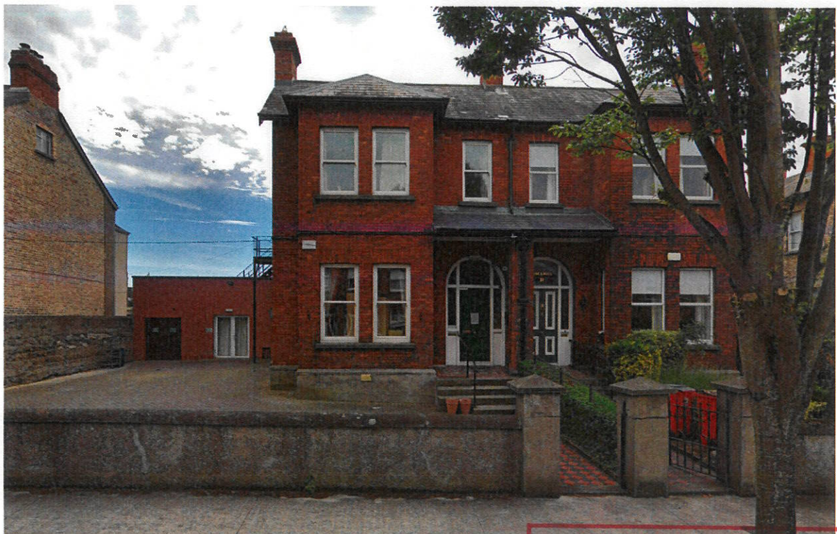
Figure 3.0 Existing front elevation of No. 30 Haddon Road, Clontarf, Dublin 3
