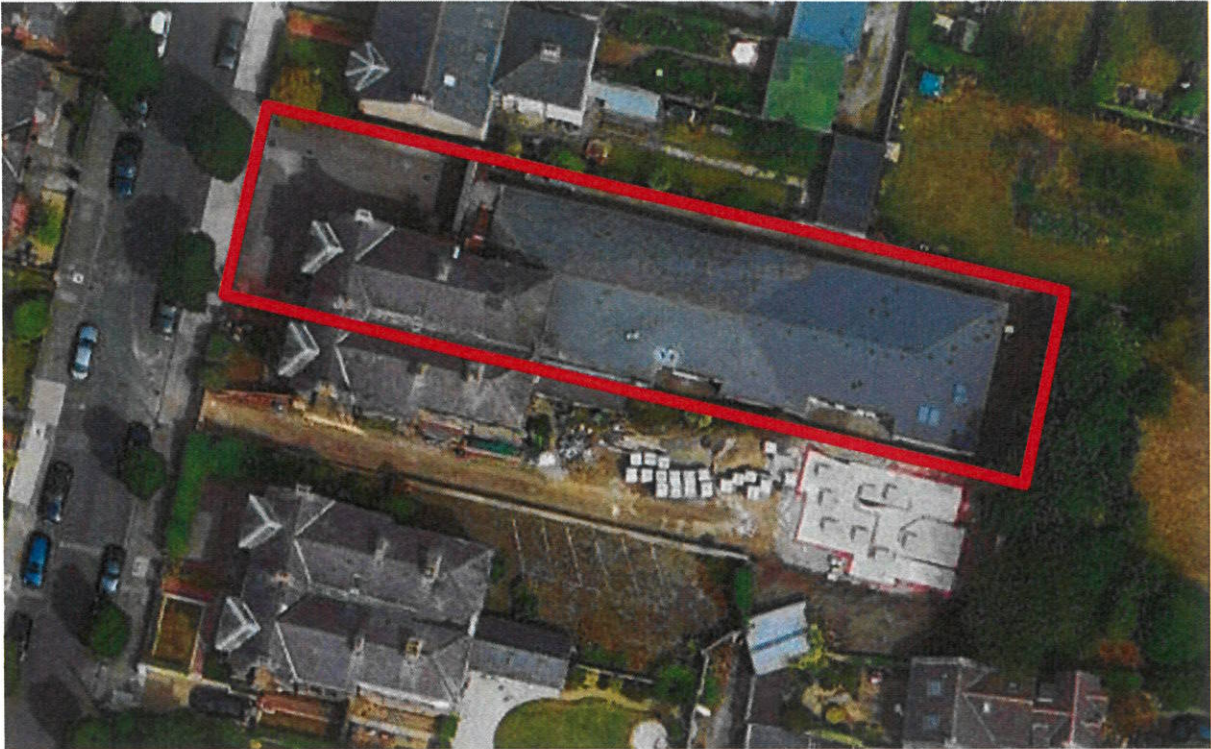
Figure 4.0 Aerial image indicating the subject site at No. 30 Haddon Road, we note that there is very little outdoor open space available to serve any future occupants.
